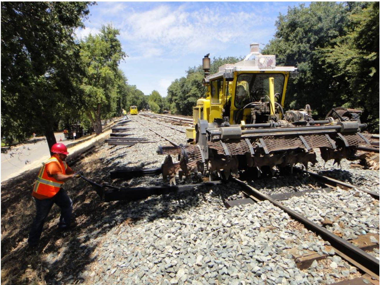
Mike H. in the scarifier/inserter and Joe insert the new ties
