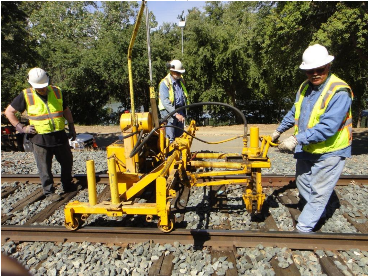
Meanwhile, on the Main, Scott fires-up the spike-puller. Fred and Alan assist.
