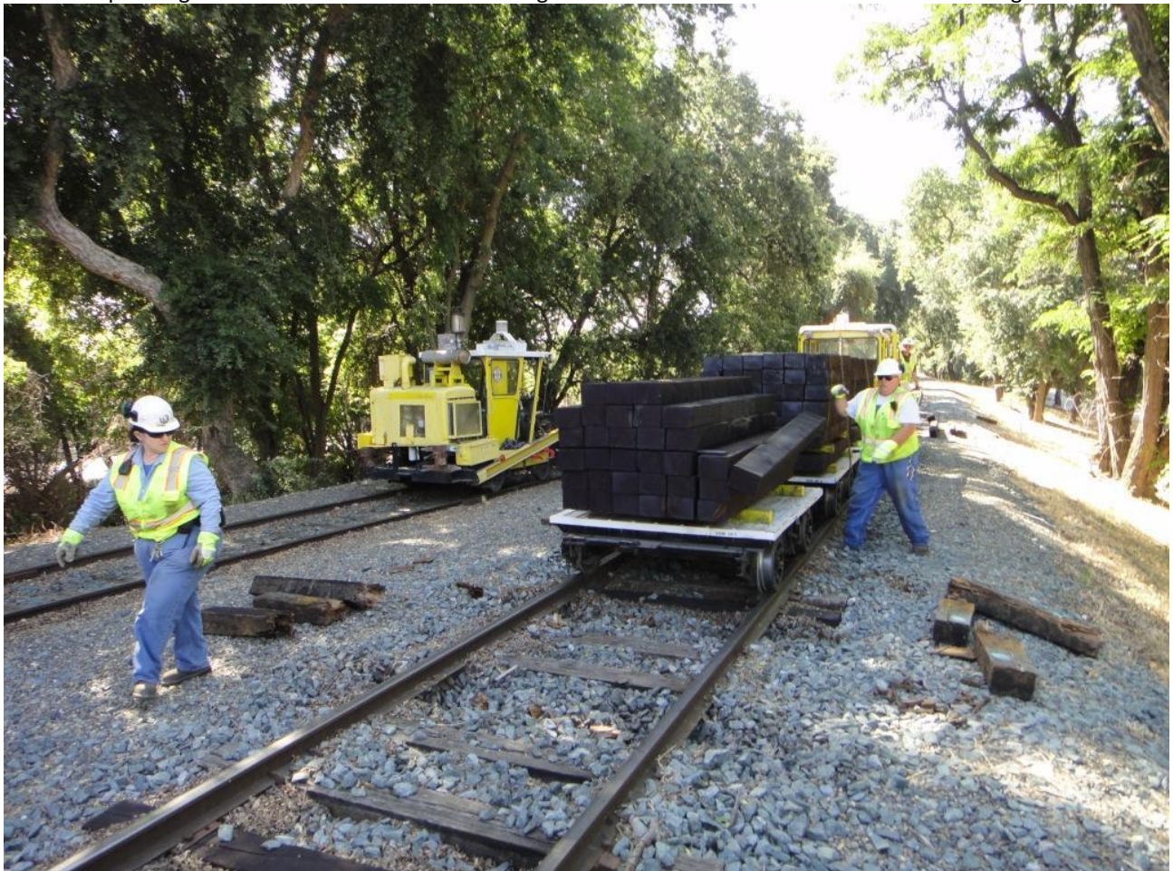
Harry and Heather follow behind the tie-shear dropping new ties for insertion
