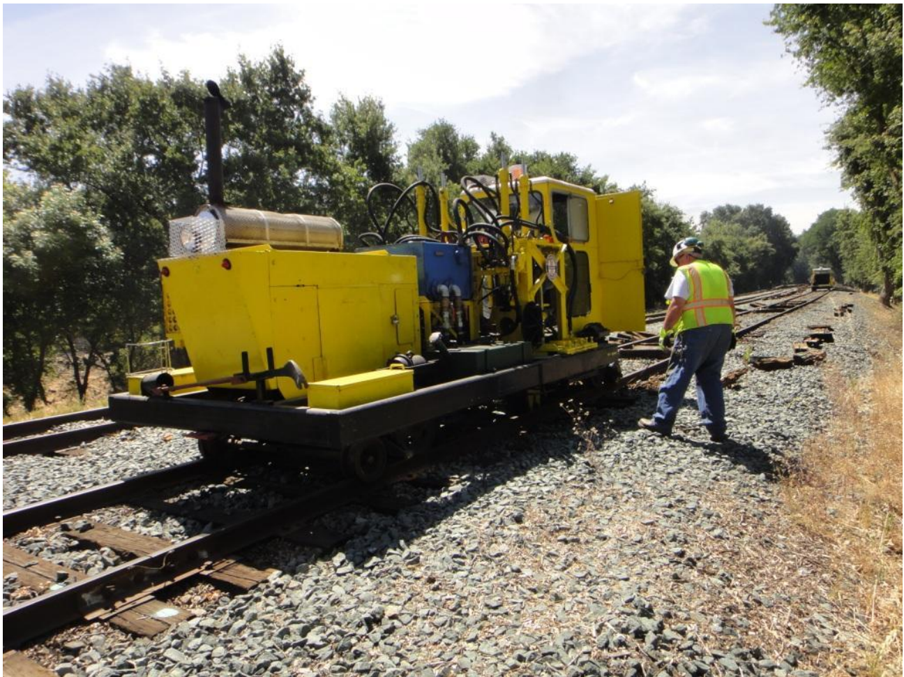
Harry guides Frank in the tie-shear as it cuts its way up the Mainline
