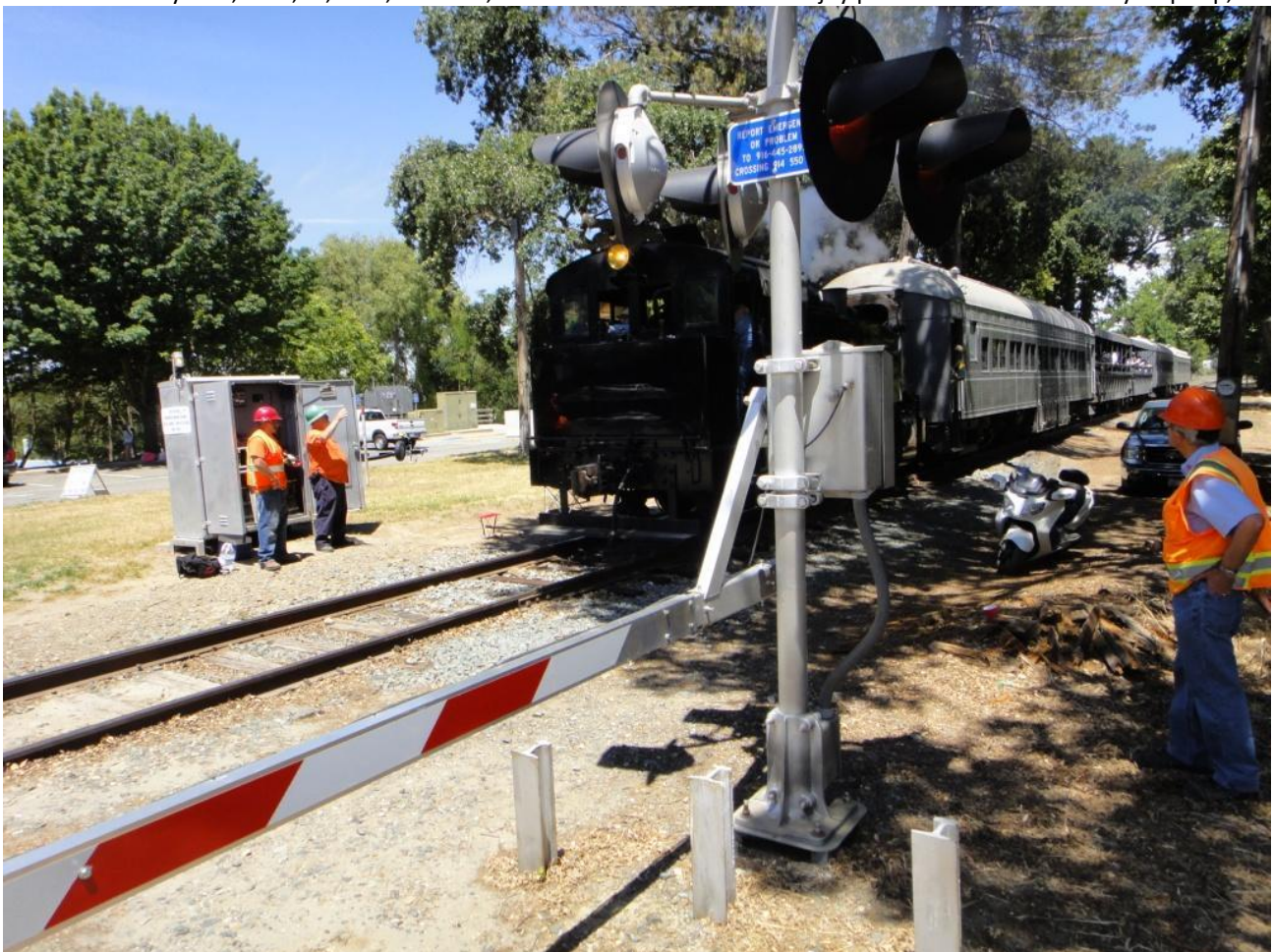
Signals Al and Dale guarantee a safe passage of the train across Front Street by manually deploying the grade-crossing warning system
