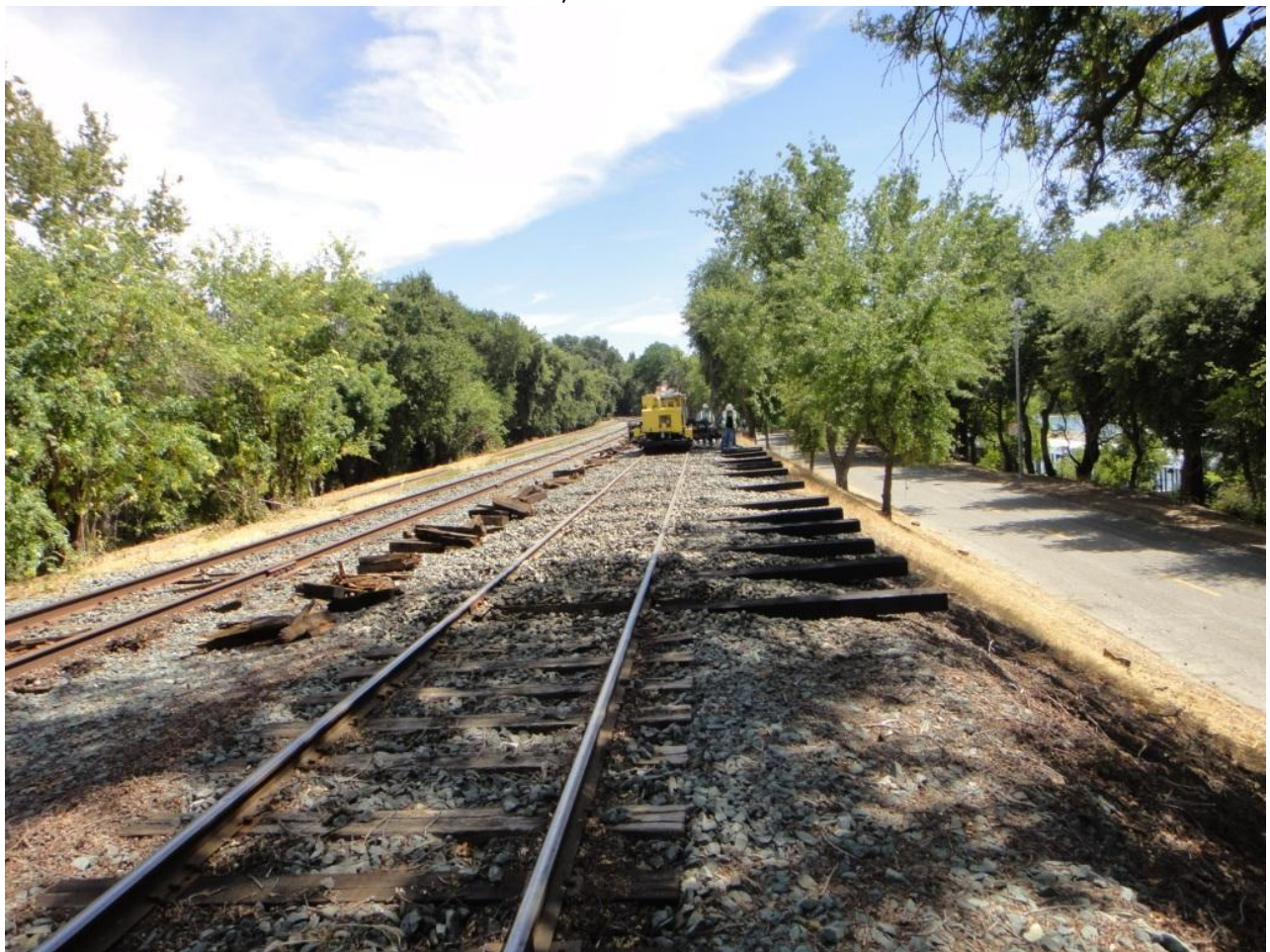
New ties ready to pull-in
