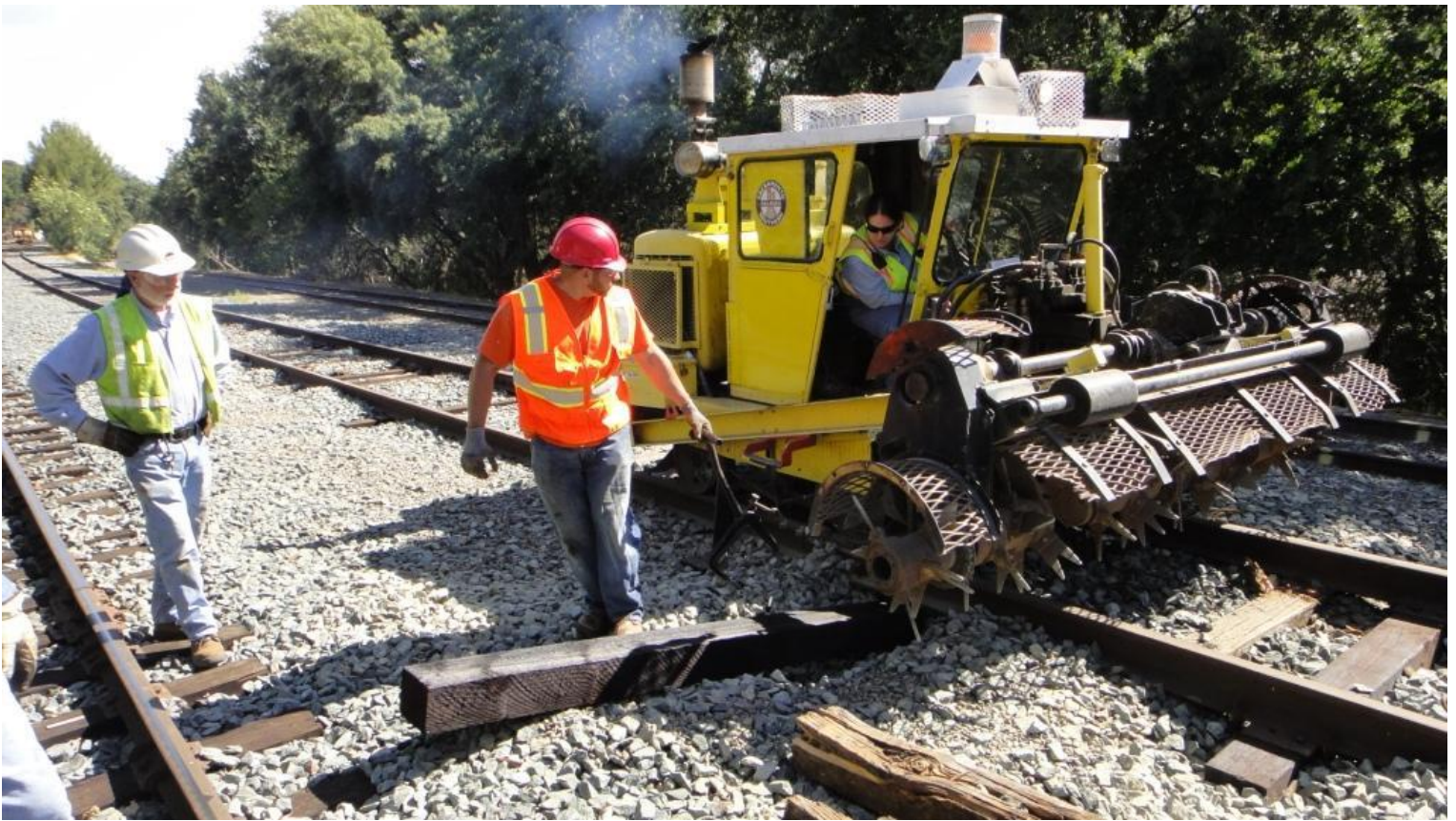
One final tie to install on the Miller Park Siding – Mike M., Joe, and Heather in the scarifier/insertor make quick work of it
